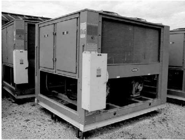
Figure 3.19 A typical air-cooled condenser ( Courtesy of Trane Company ).
